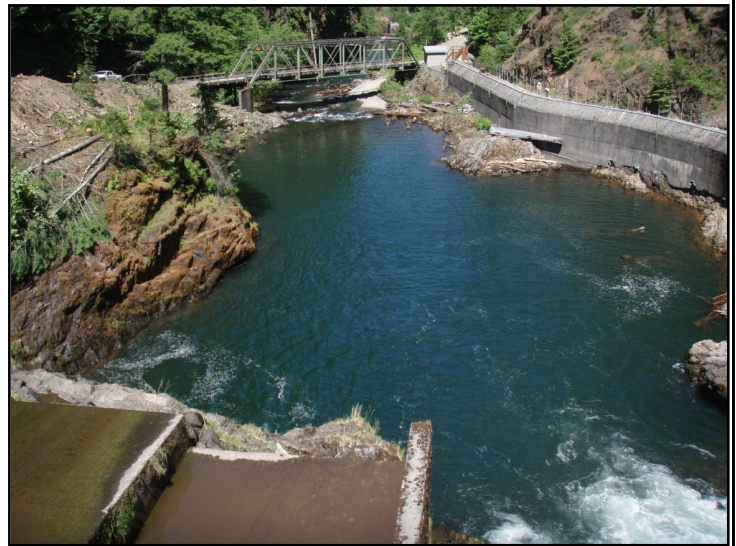
North Umpqua River viewed from Soda Springs dam prior to dewatering on day 1 (6-21-10 0800). Photo:R Grost
